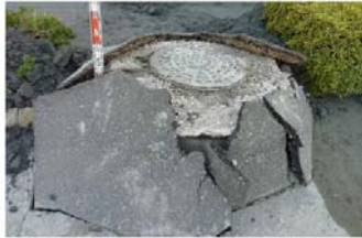
Urayasu city: liquefaction and floating of a manhole
