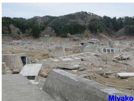
The 10m-high tide embankment was destroyed in Tao district, Miyako city, Iwate prefect.
