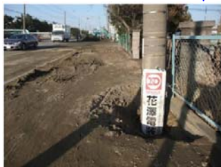
Around Chiba port: Subsidence of a electric pole and large volume of sand boil
