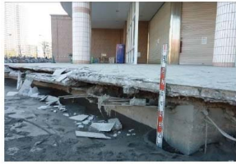
Urayasu city: Lifting of building basement due to liquefaction and subsidence
